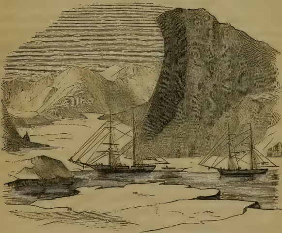
ADVANCE AND RESCUE IN BARLOW'S INLET.
